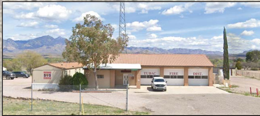
2227 I-19 Frontage Rd.
